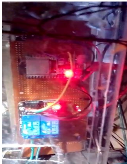
Gambar 9. Modul Relay 2 menyala pompa off exhaust on
